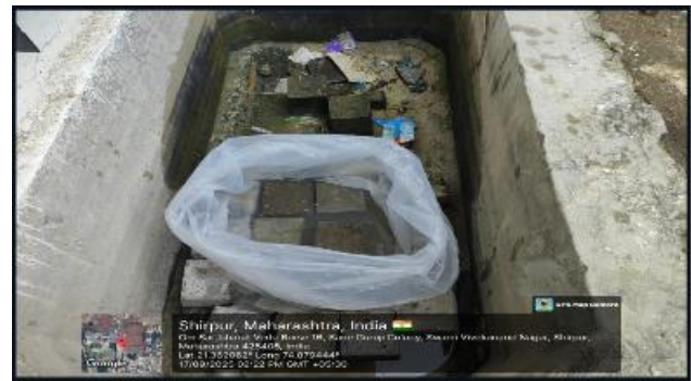
Fig.2 Curing of M40 Grade Cubes
