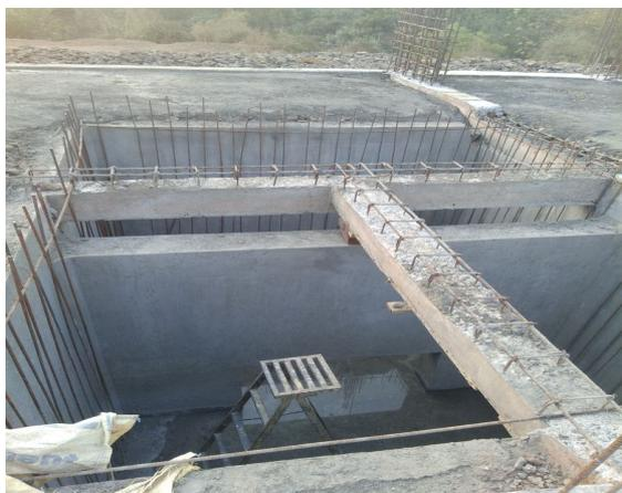
**Fig 7.3: Photo. Plinth Beam passing through Septic Tank**
