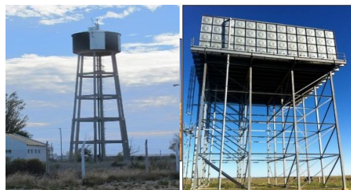
Fig: Different shapes of elevated water tank
