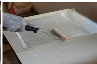
Fig. 1.2: levelling with roller
