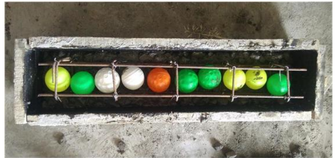
Fig. 3. Bubble lattice placed in concrete
