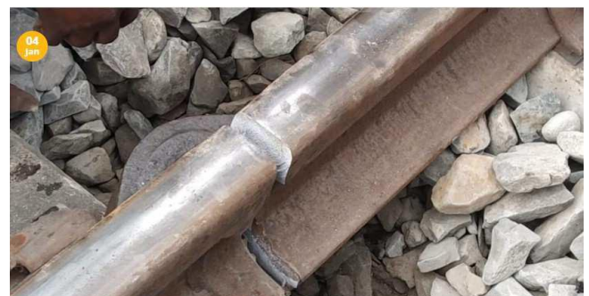
Fig. 2 Part of the track which was has a Crack
